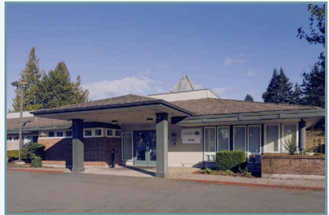
Aurora Oaks Enhanced Shelter
